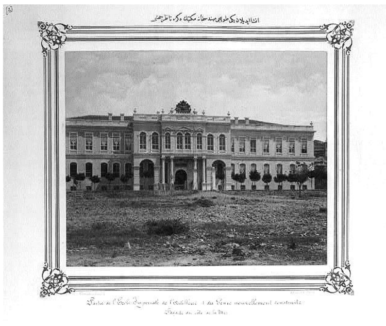
Abdullah Frères, View of the side facing the sea of the artillery engineering school (Imperial School of Artillery) which has been recently constructed, Albumen print, c.1880-1893, LOT 9542, no. 2
